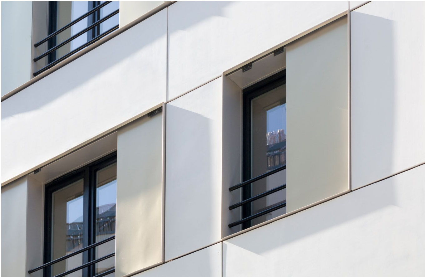
Apartment block, France, 2017 - Philippon - Kalt Architects & Fehr
