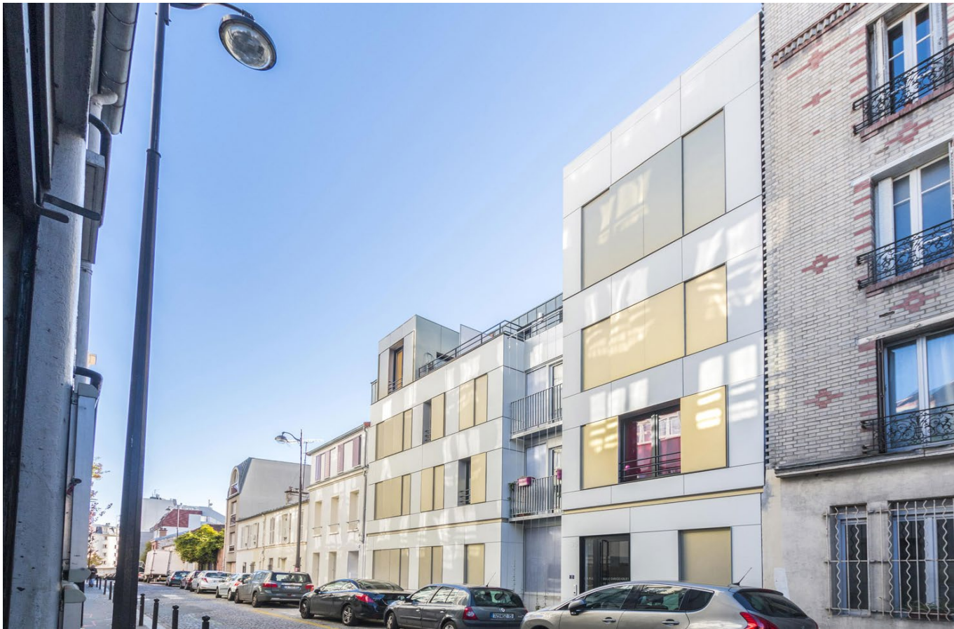
Apartment block, France, 2017 - Philippon-Kalt Architects & Fehr
