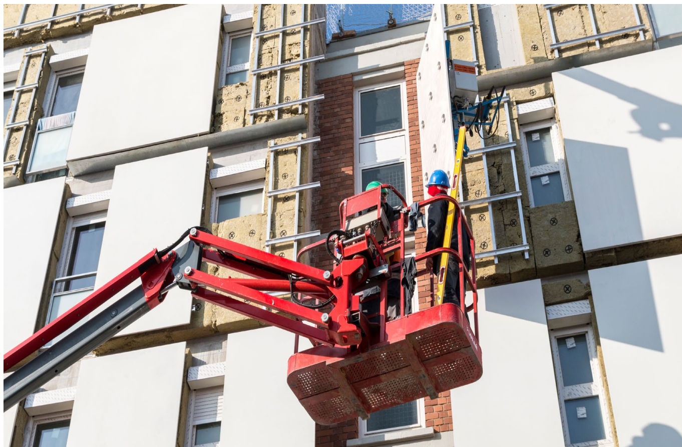
Chaperon vert, France, 2017 - AEC Architecture & Fehr
