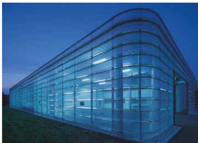
Bâtiment industriel Steba, Ottwang (A) Architecte: Arch. Dipl.-Ing. Ivo Kux
